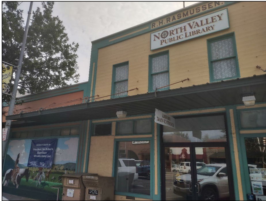
Photo 1. July 29, 2024. Outside looking northeast: Front entrance for the North Valley Public Library, a combination of three buildings plus an addition on the alley side. The main entrance is located on the yellow two-story building. The orange and red painted building is part of the library. The building's age ranges from 1910 and 1940; a remodel with an addition was performed in 1960.
